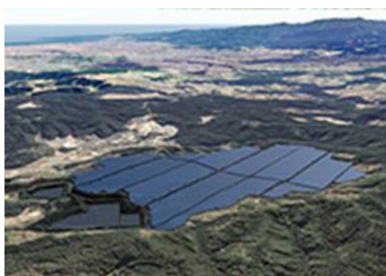
Pacifico Energy Hosoe Mega-Solar Power Project
