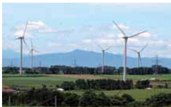
Solar and wind power projects
