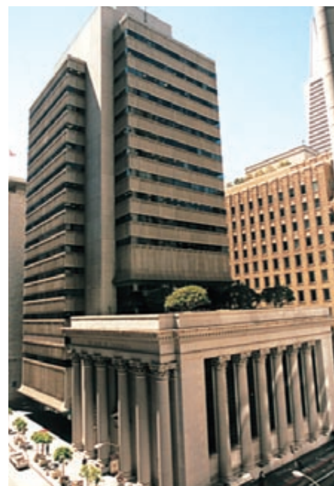
Union Bank of California headquarters
