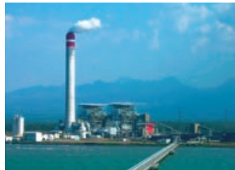
Power Plant in Central Java
