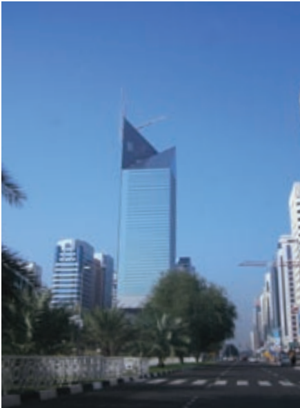
NBAD Tower, the location of the Abu Dhabi office
