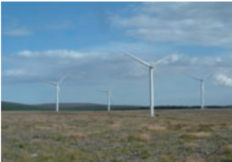
Crystal Rig Wind Farm
